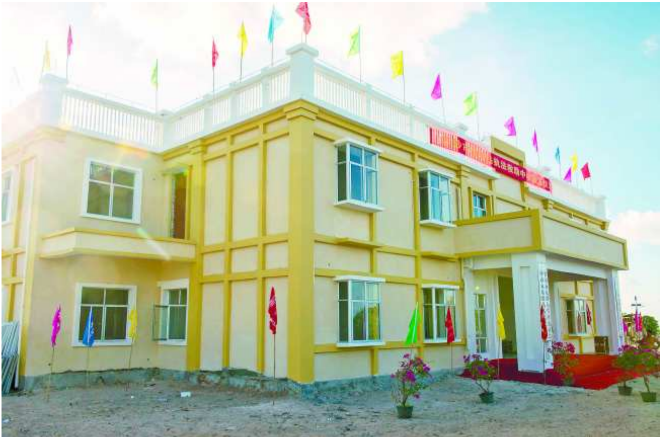
28 July 2016: Drummond Island finishes construction of its PAFD and militia outpost multipurpose building. ( Macao Daily )
