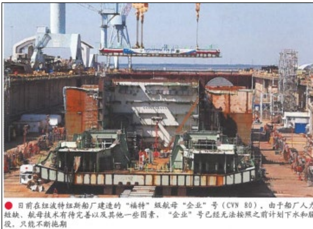
A Ford-class aircraft carrier, the USS Enterprise (CV 80), currently under construction at the Newport News Shipyard. Due to shipbuilding manpower shortages, needed aircraft carrier technical upgrades, and other factors, the USS Enterprise could not meet its planned launch and commissioning dates, which have been constantly pushed back.
