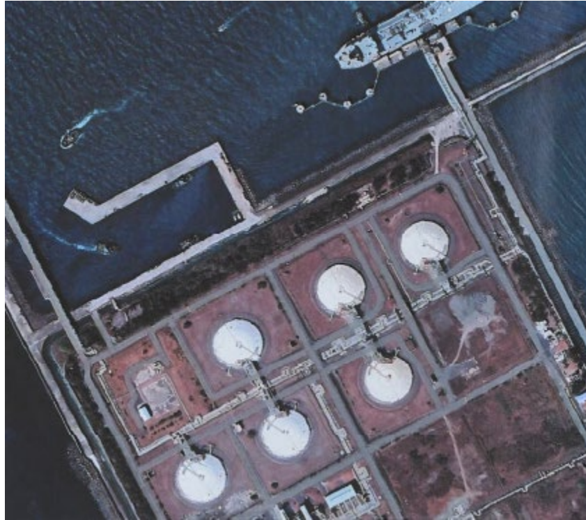
Taiwan's first liquid natural gas terminal—referred to as “Terminal 1”—is located in the Yongan district of Kaohsiung city. With a total storage capacity of 4.5 million tons, it is the largest liquefied natural gas terminal on the island.
